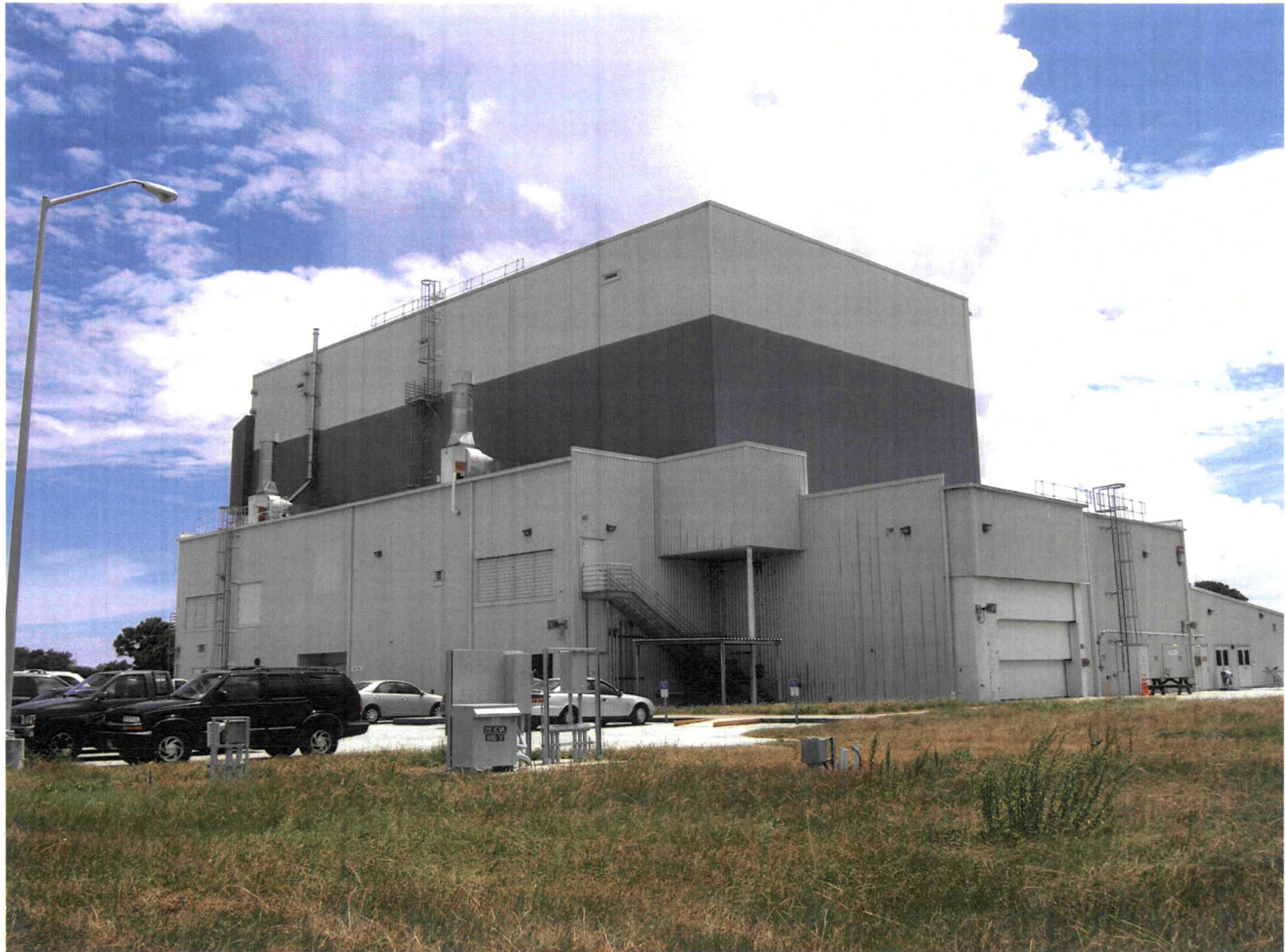
Figure 1. Multi-Payload Processing Facility (MPPF)
